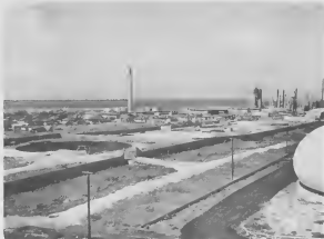
THE GROUND is cleared and bottoms are ready for the erection work to begin. This sequence of photographs shows construction progress on a E SUELO ta wòrdè limpí i prepará pa e trabao di erección cuminsa. E sucesión di retrato aki ta muntra progreso di construcción ariba hen-
